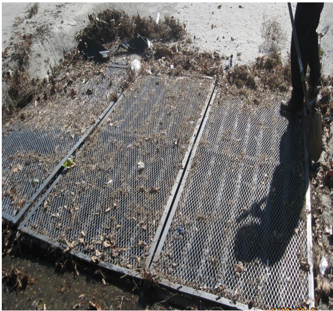
(Above) Victoria Inlet Being Cleaned (Below) Victoria Inlet Missing Mesh Panel
