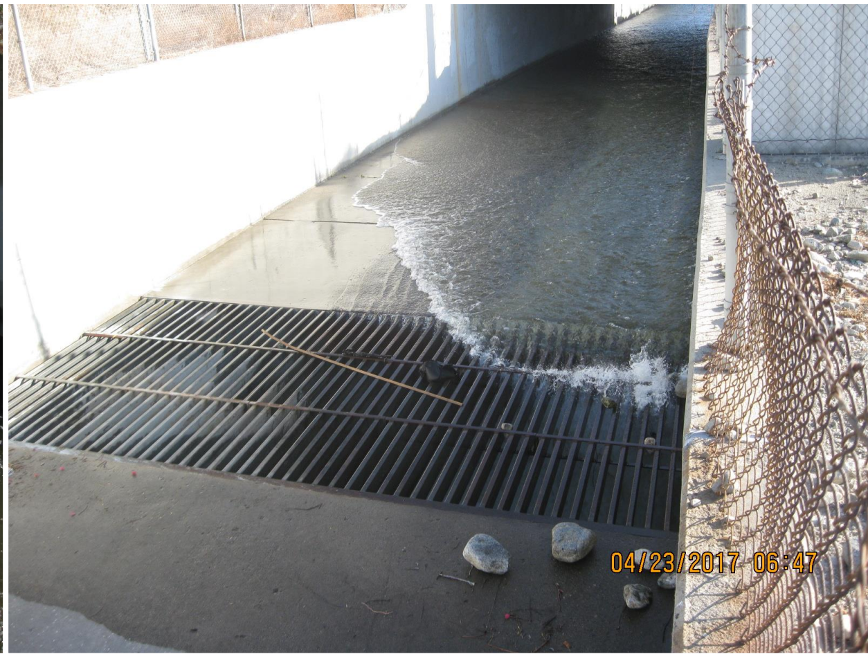
Approximately 60 CFS flow into Montclair 1 Inlet
