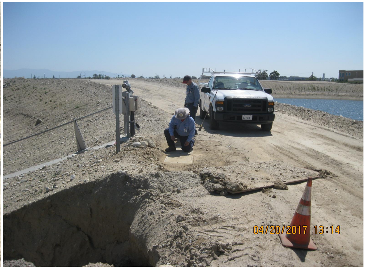
Inspecting Communication Wire Pull Box, note erosion in road
