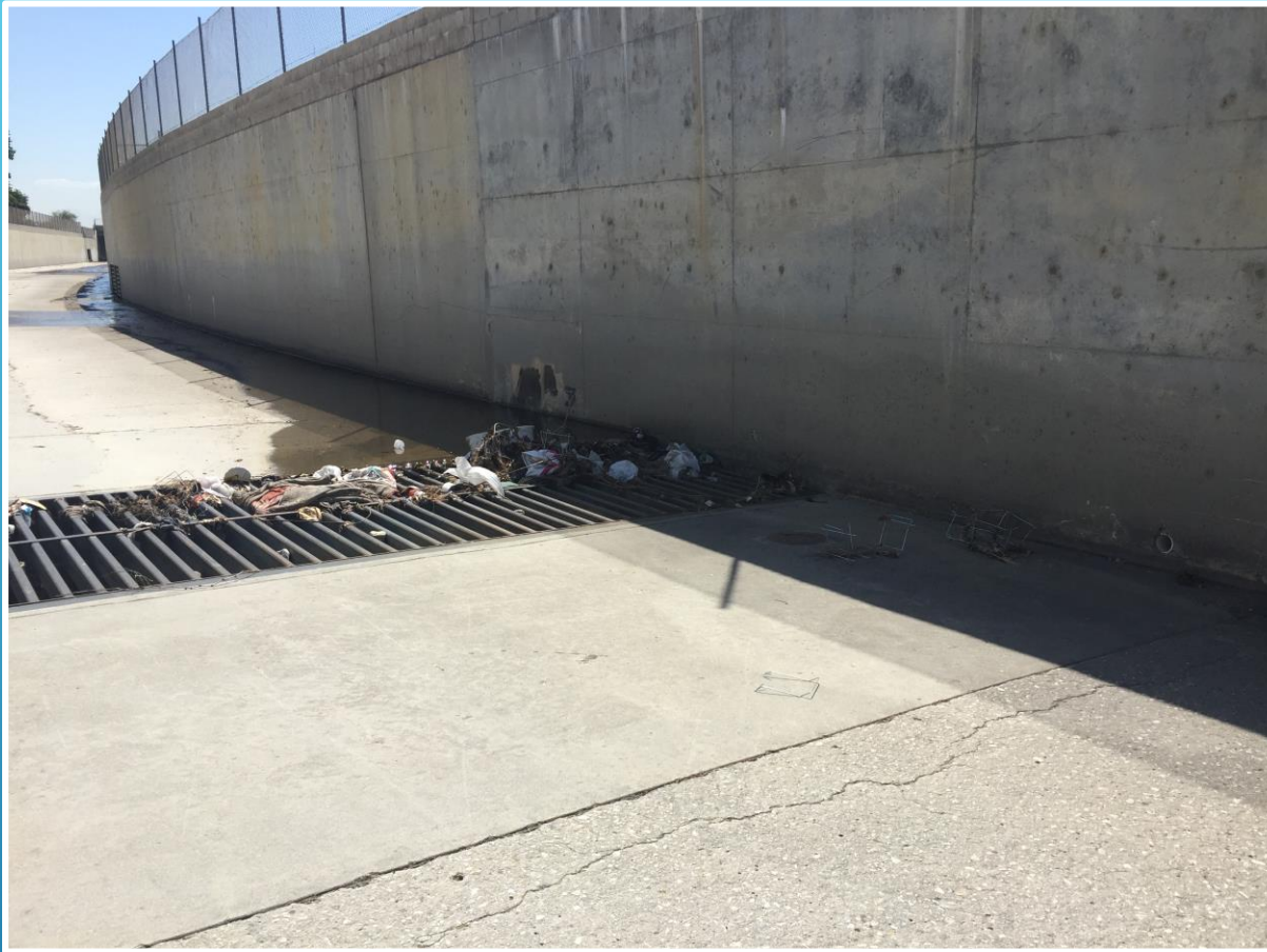
Trash Buildup on Grate Leading to Turner 4A
