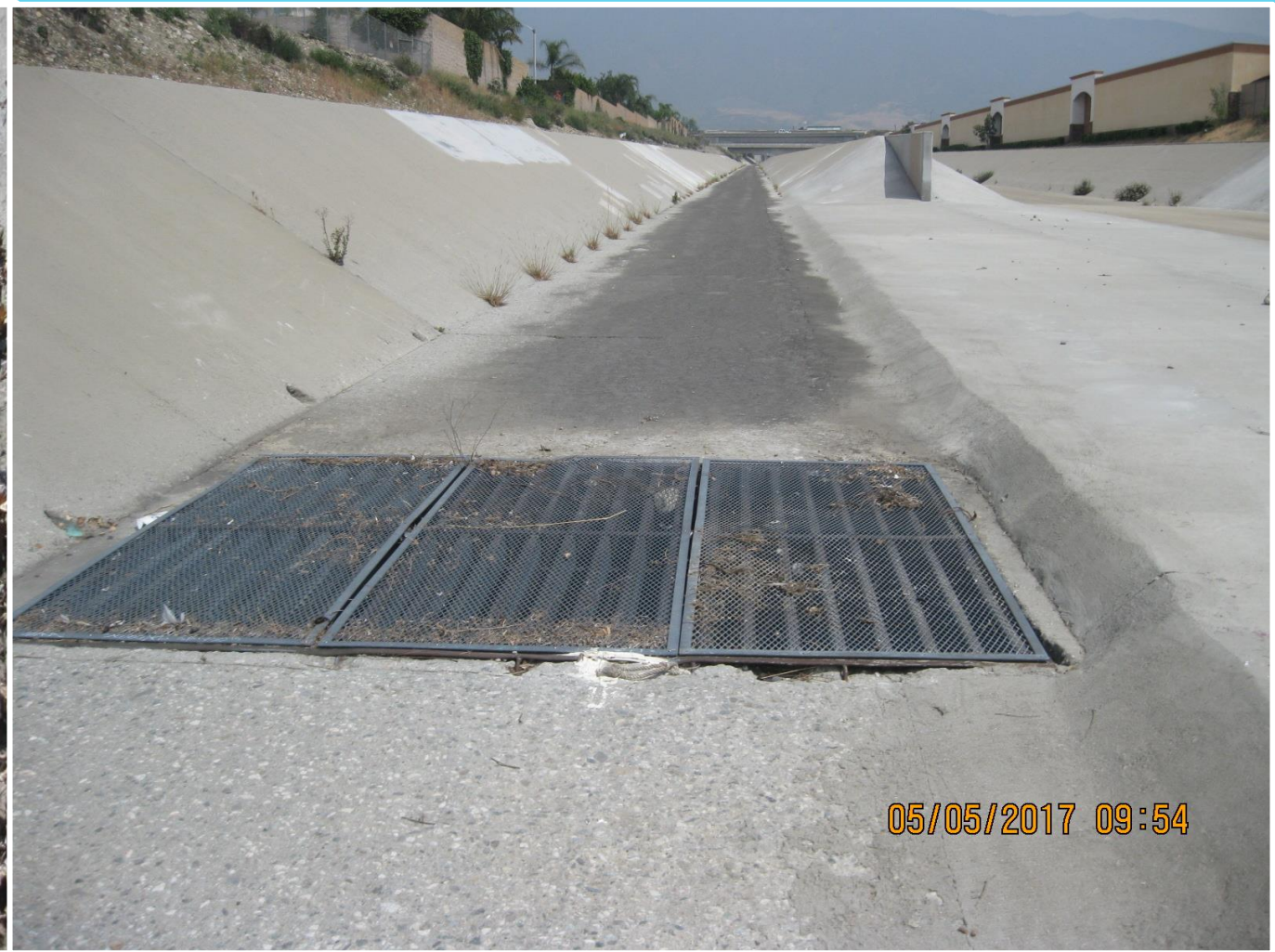
Victoria Inlet Mech Panel Reinstalled
