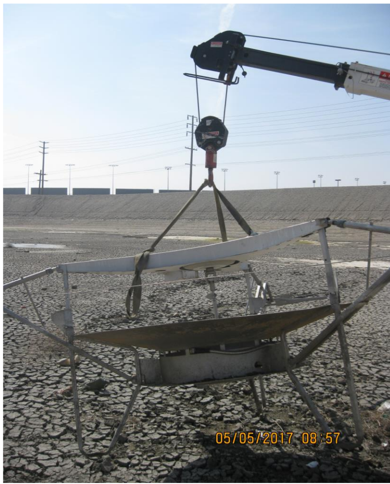
Solar Bee Main Frame Being Hoisted
