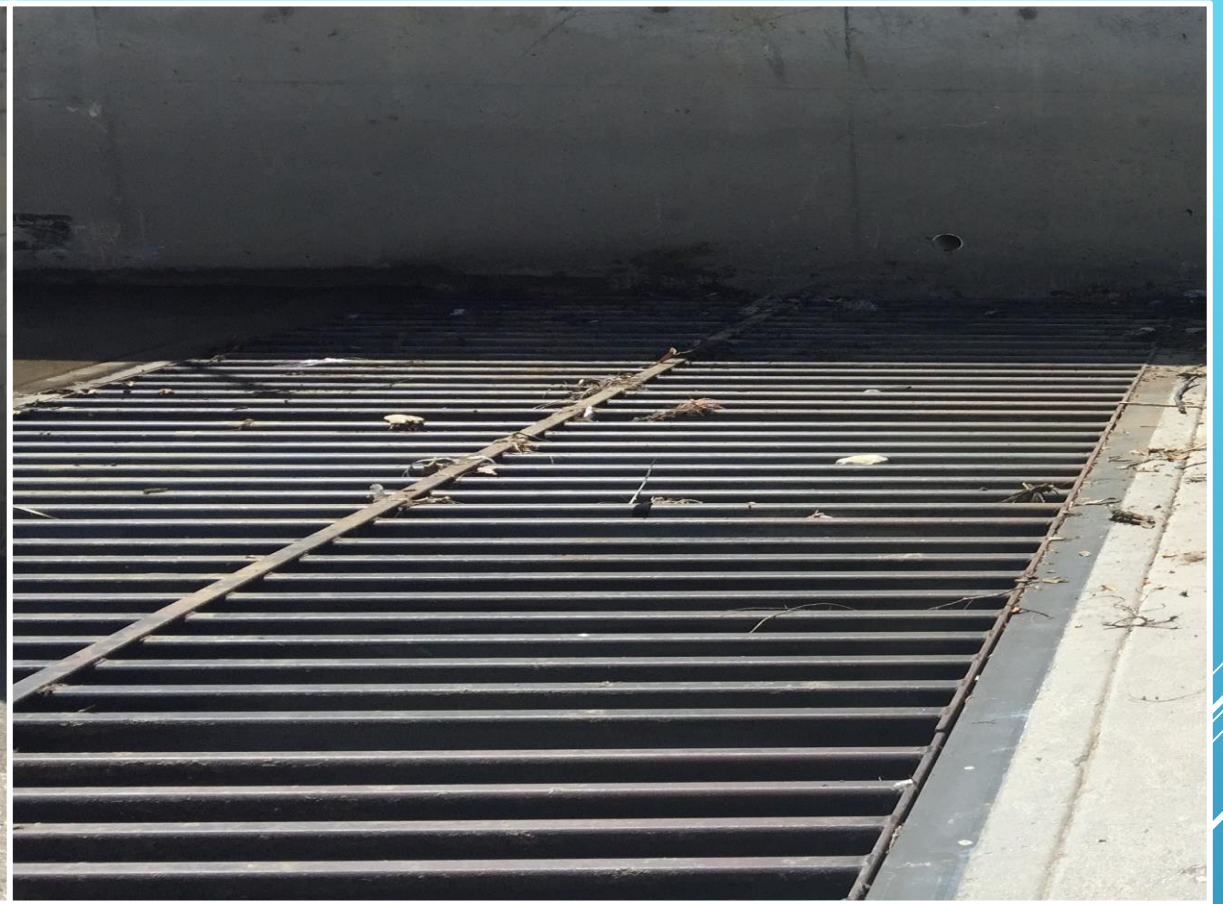
Turner 4A Inlet Cleaned of Debris
