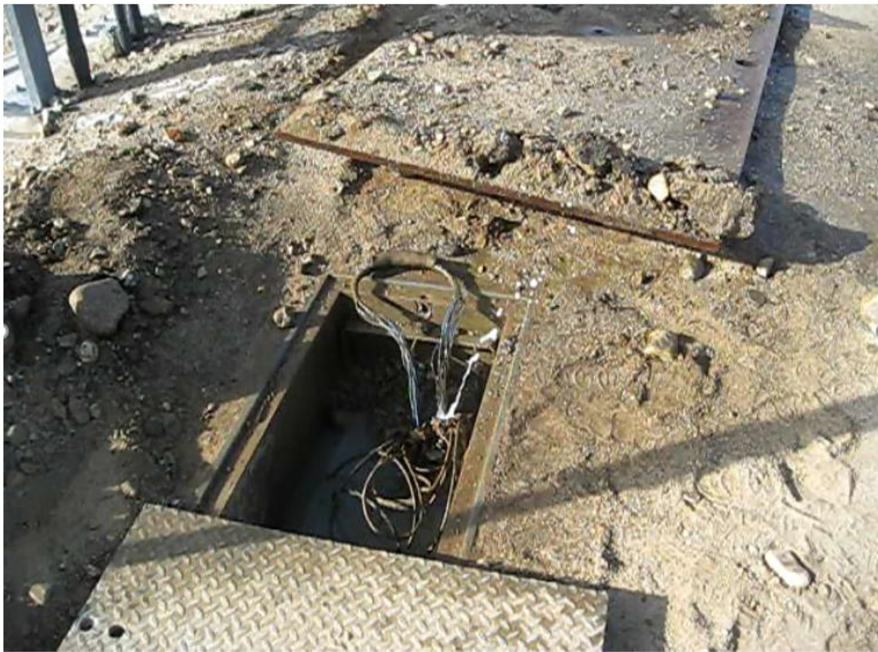
Pushing water Out of Communications Conduit at Turner 4A
