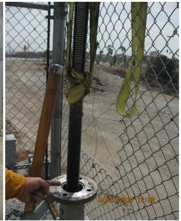
College Heights West Inlet Valve Manual Open for Imported Water
