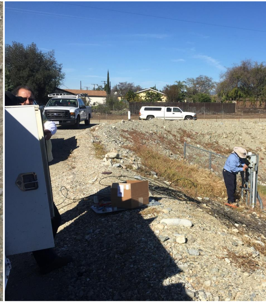
Final Wiring Montclair 1 Level Transmitter
