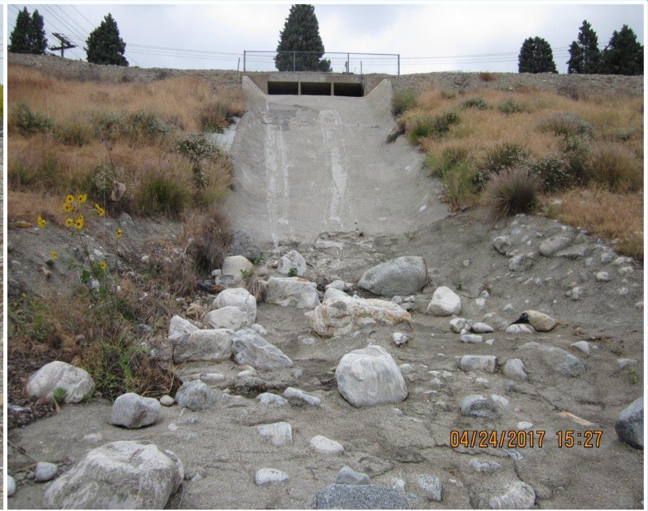
No Seepage Evident from Montclair 2 Spillway with High Water at Montclair 1
